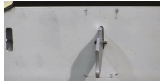
3 Engage the rafter bracket into the slot provided on the ridge.
