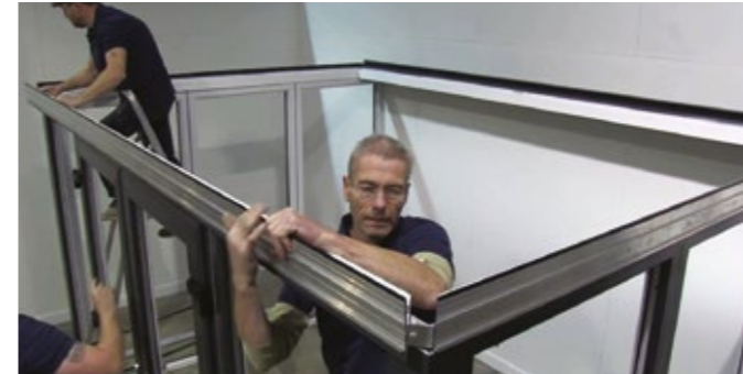
7 Lift the final front ringbeam into position and slide the ringbeam bracket into the channel on the
