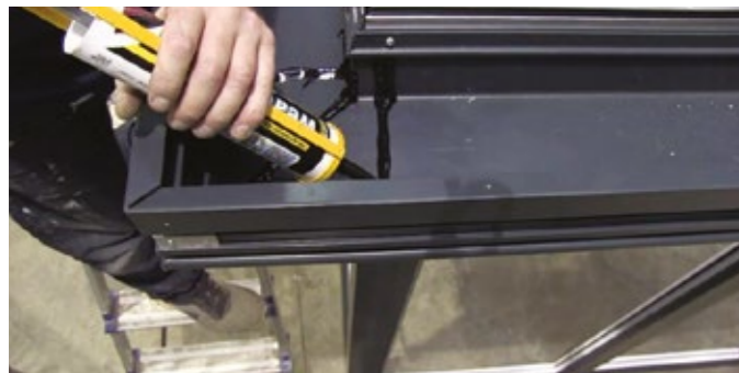
16 Cover the inside of the aluminium box gutters at the corners with sealant.
