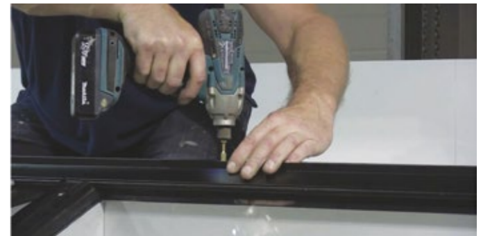
4 Fix the ridge pressure plate centrally to the main ridge body with screws.
