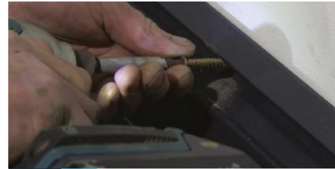
9 Fix the box gutter securely to the rear wall (see Figure 1).
