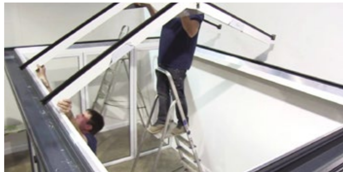
10 Lift the main A-frame into position.
