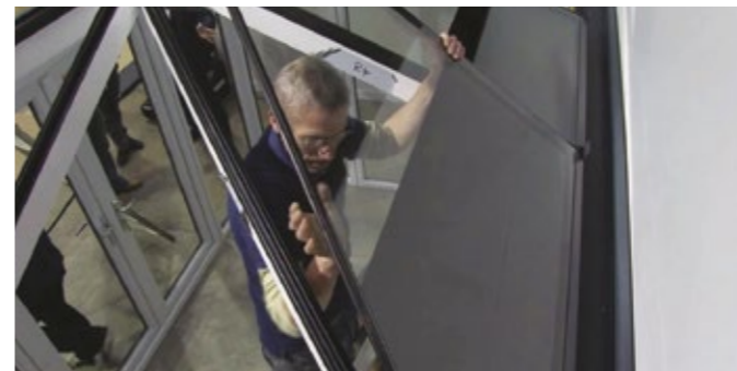
5 Fit all the rear units of glass keeping the glazing end closer between the rafters.
