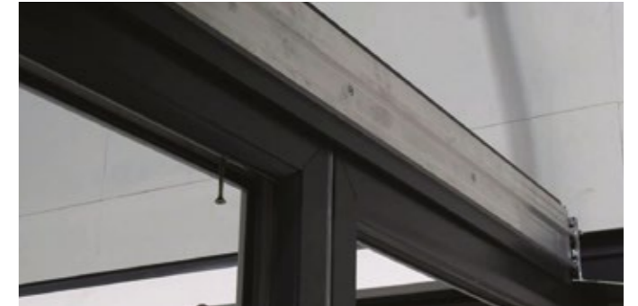
8 Fix the ringbeam to the window frames around the perimeter of the Skyroom roof.
