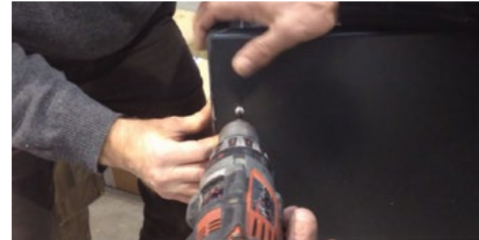
7 Drill the top mushroom screw through the cornice into the bracket held at the back of the cornice.
