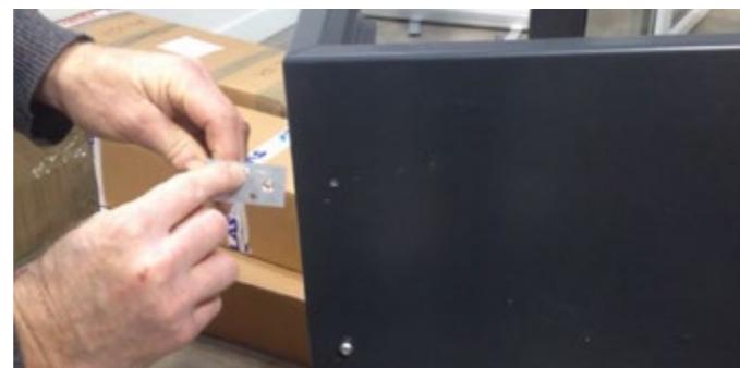
6 Screw the bottom mushroom screw through the semi-drilled holes in the cornice. On the top hole line through the smaller hole on the bracket internally with the drill hole on the cornice.
