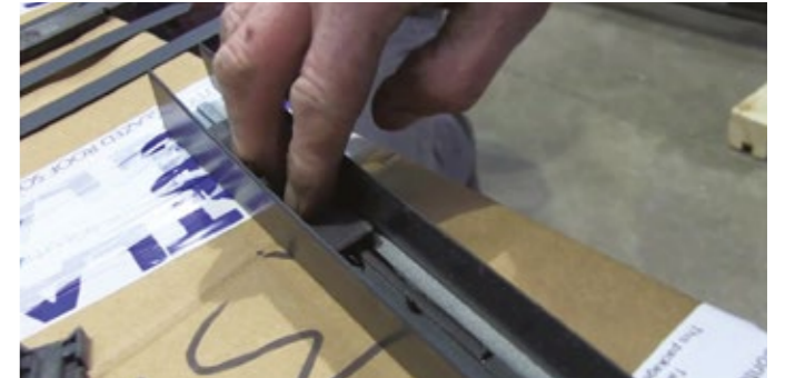
2 Glue packers into place at bottom glass end closers.
