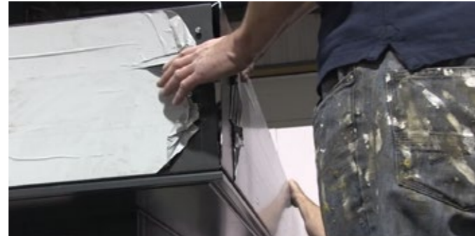
2 Fit remainder of cornices.
