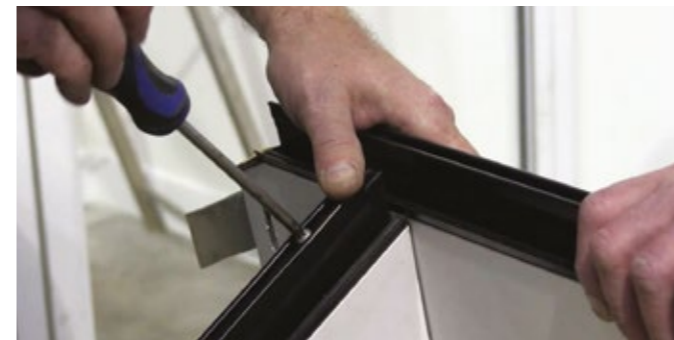
5 Screw into position by fixing the top screw.
