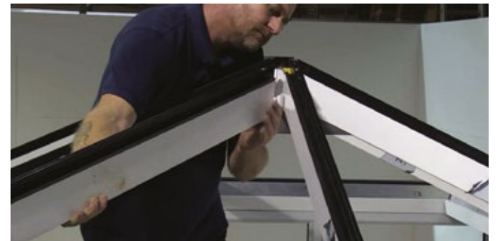
4 Slide the hip rafter over the bracket and push it tight against the ridge.
