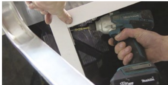
3 Screw through the angle brackets into the side of the rafters.
