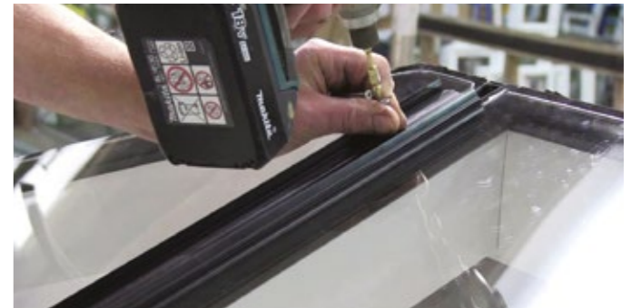
2 Fit remaining pressure plates into position.
