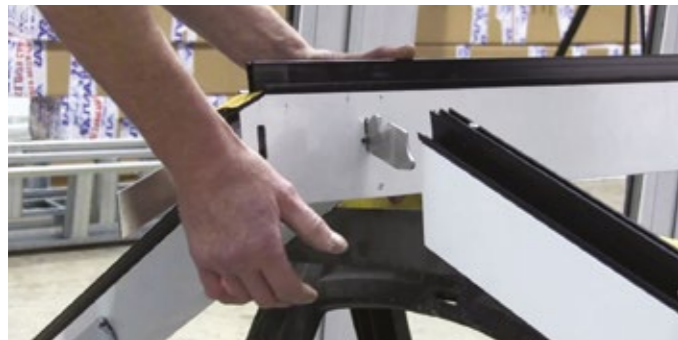
9 Fix remaining rafters on the main A-frame.
