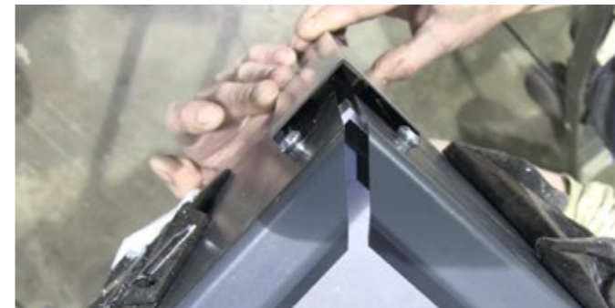
9 Slide the finishing corner cornice angle over the mushroom screws by sliding them up from below.
