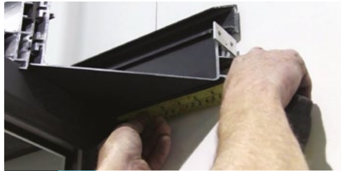
4 Centre the gutter on the frames.
