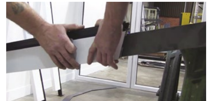
6 Slide the adjacent rafter over the steel angled bracket.
