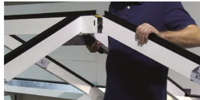
3 Fix the opposite ridge end rafter.
