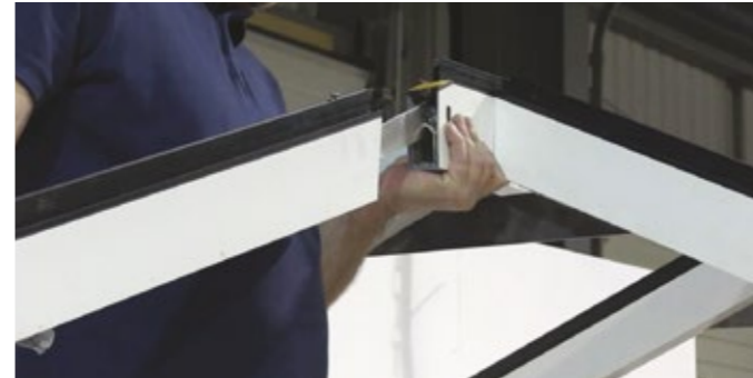
1 Slide the ridge end rafter over the pre-fixed ridge bracket.
