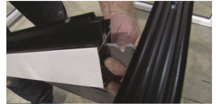
4 Slide the rafter over the bracket, making sure it locates in the central bracket channel.
