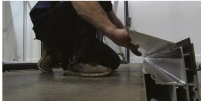
2 Remove the ringbeam flaps from the ringbeam.
