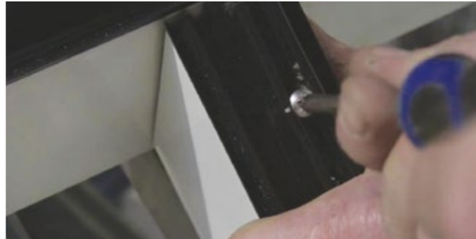
8 Screw into position by fixing the top screw.
