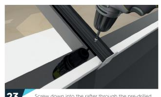
Screw down into the rafter through the pre-drilled holes in the pressure plates using the 4.2 x 45mm screws. Repeat for all the rafters.
