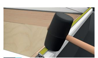
Fit supplied glazing support trim between rafters and tap on with a rubber mallet, then silicone foamboards to the ringbeam flap between the rafters.
