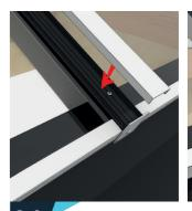
Fit all the rafter topcaps according to the correct cut length and roof plan position. Locate over the top of the pressure plate and push down. A rubber mallet may be required.
