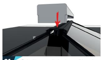
Fit the ridge top cap in place by centralising and applying pressure from one end to the other. A rubber mallet may be required.
