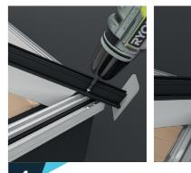
Fix hips into ringbeam using the provided 4.2 x 25mm fixings on either side of the rafter as shown.
