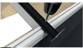
Check that the rafter is square to the ringbeam. Fix the 4.8 x 50mm screw supplied centrally through the bottom of the transom rafter as shown to secure the rafter.
